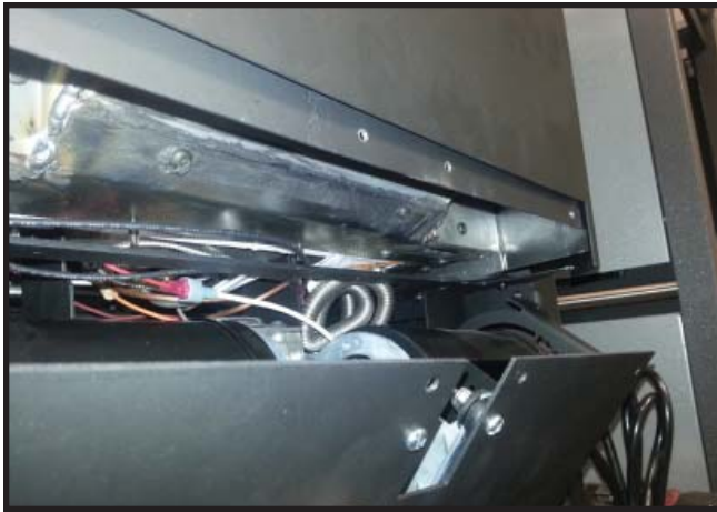
13. Screw the fan assembly to the appliance: 2 screws (1 each side) into the firebox bottom.
