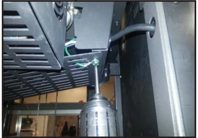
Screw in remaining 3 screws to fasten wire cover.
