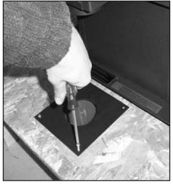
Using the supplied screws, secure the floor flange to the floor or wall at this time. Slide the 3" flex tube onto the adapter and secure with enclosed hose clamp. Run the 3" flex inside the 6" galvanized pipe secured earlier.
