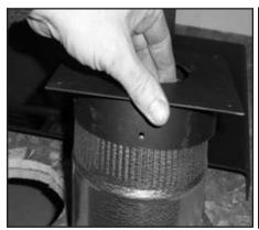
Included with this kit is a 24" length of 6" galvanized pipe. You can attach the pipe at this time if the access under the floor is limited. Use the enclsoed #10 x 3/8" sheet metal screws to make the connection secure.
