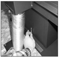
For mobile home applications please anchor the stove using the enclosed 3" lag screw with 1/4" washers. The approved location, as shown here is located at the rear of the stove. For added safety, remove ash pan and drill a second 1/4" hole near front of the base. A second 3" lag screw has been included for this purpose.
