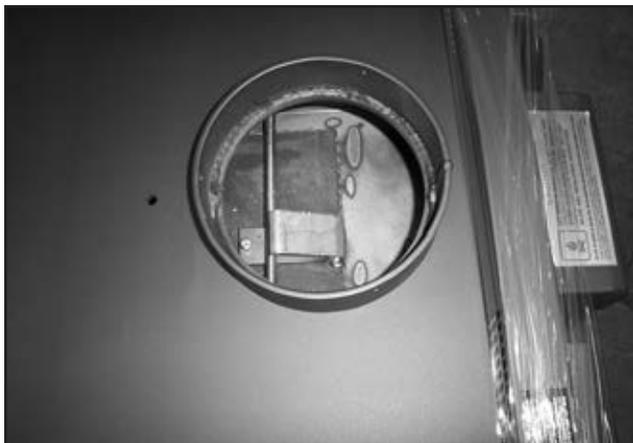
Although this photo shows a new style bypass plate installed, the old style (short ramp) will be in this position when you lift the pipe off the top of the stove. You will find it necessary to move the bypass rod to make removal easier. This can be done by moving the bypass handle on the side of the stove.
